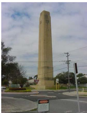
An art deco tower built in 1941 to vent sewage fumes into the atmosphere. The tower is 38 metres tall and the second tallest sewer vent in Australia. Inadequate design led residents to complain of unpleasant smells, particularly during certain weather conditions. The base of the tower was cemented over to render it non-functional. The tower was referred to as *Dumas' Folly* after the engineer RJ Dumas.
